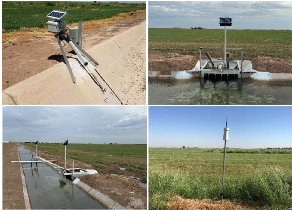
Figure 1. Automated surface irrigation infrastructure utilized in forage production fields in Imperial Valley, California, including solar-powered automated canal gates and real-time water advance sensing stations. The system regulated irrigation inflow based on field water advance conditions to improve irrigation efficiency, reduce tailwater runoff, and optimize surface irrigation management.
