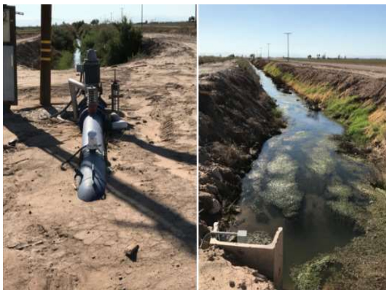
Figure 3. Tailwater recovery infrastructure utilized in forage production systems in Imperial Valley, California. The system captures irrigation runoff through agricultural drainage channels and recirculates the recovered water back to irrigated fields to improve irrigation efficiency, reduce operational water losses, and enhance on-farm water reuse under low desert conditions.
